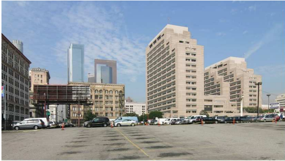
Reagan Office Building
